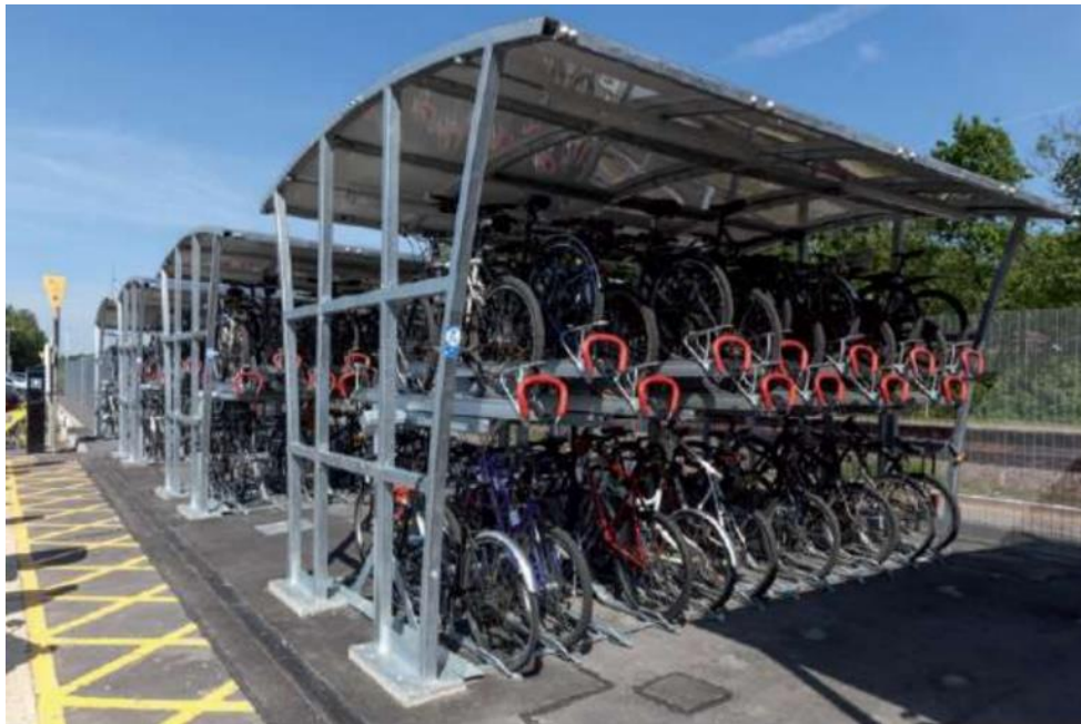
Hinchley Wood Cycle Stands - The construction of a 20-bay cycle shelter to promote ‘first and last mile’ low carbon sustainable transport options for residents and out of area commuters, travelling by train.
